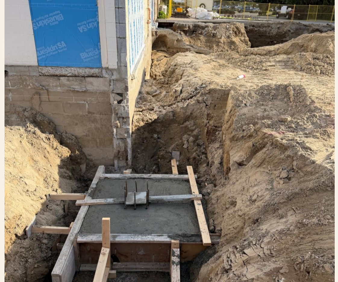
Excavation and formwork for the new structure
