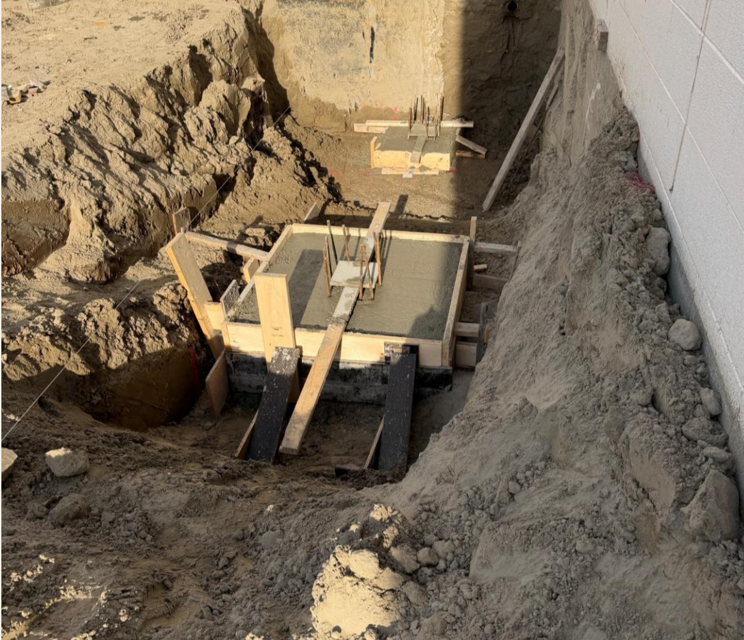
Base preparation beside the existing building
