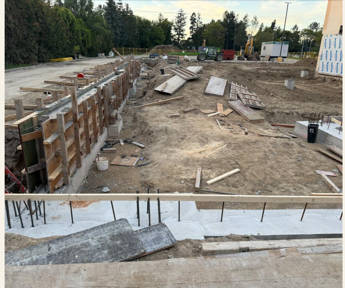
Foundation work along the west wall
