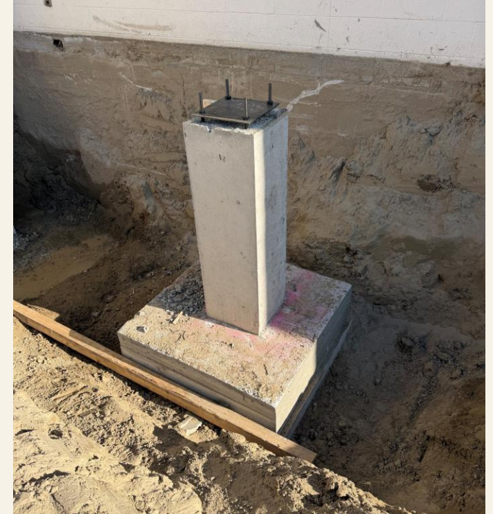
Pillar for the metal structure
