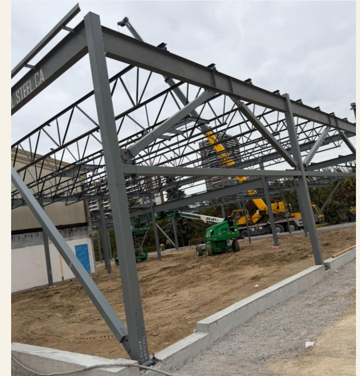
Roof trusses added to the structure
