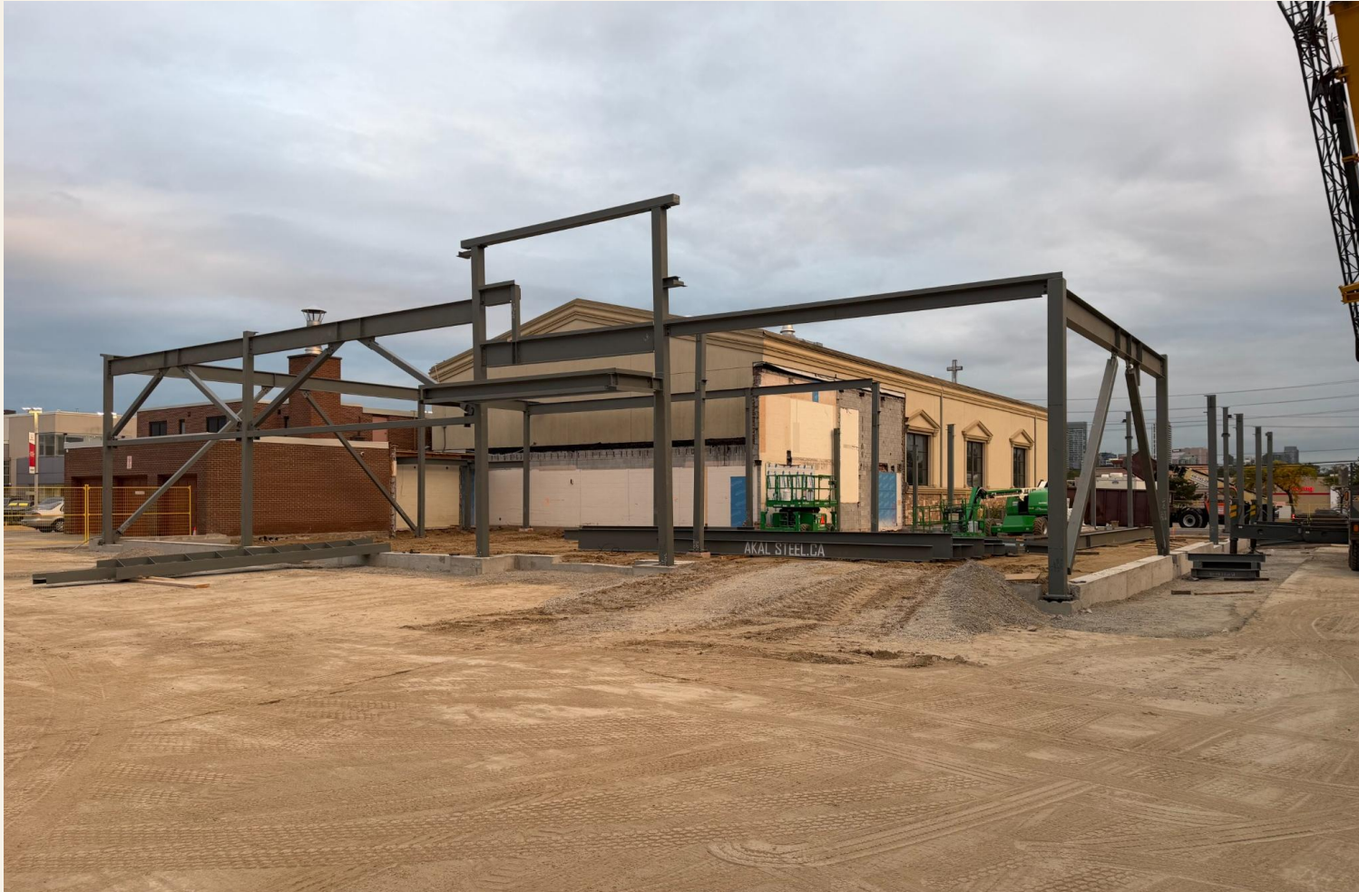
Early steel columns and beams
