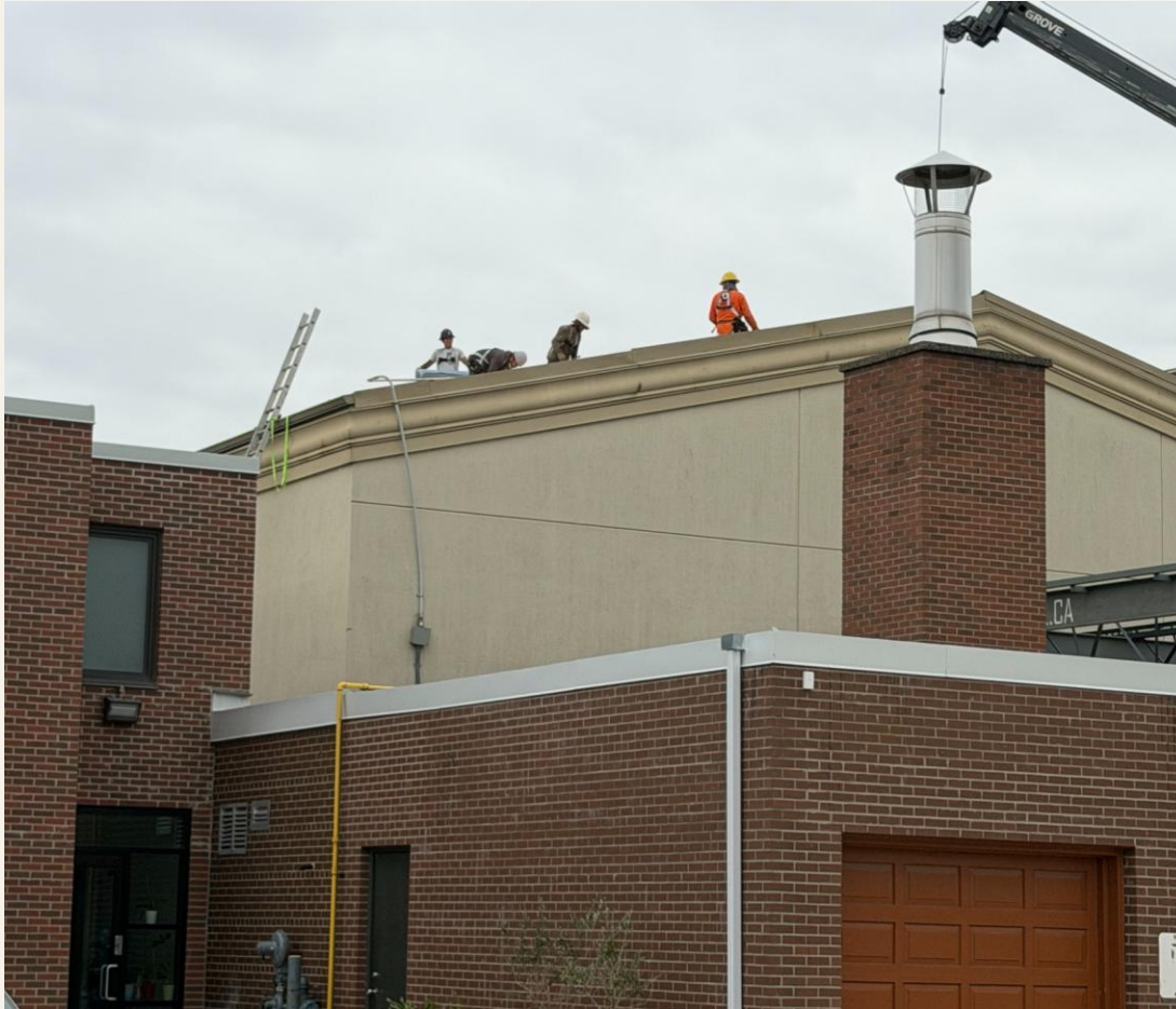
Crews working along the roofline
