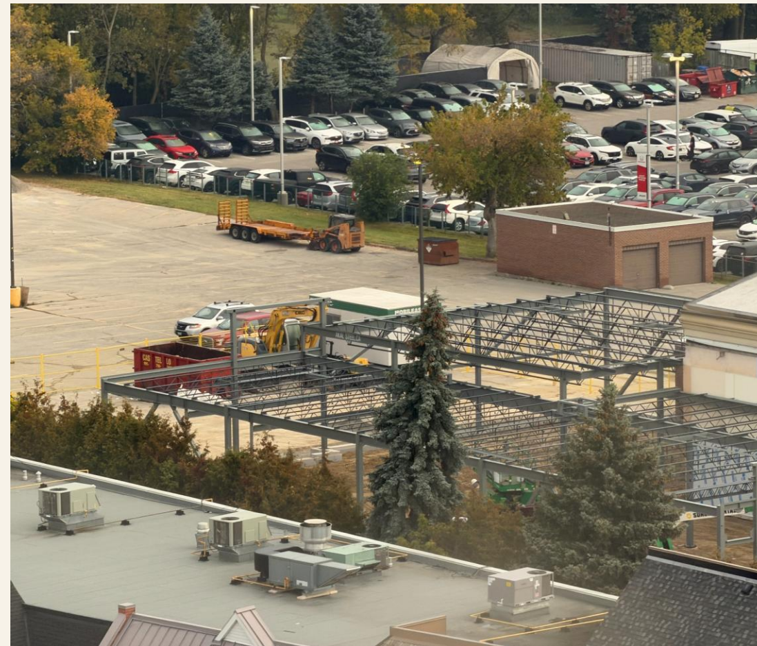
Aerial view of the expanding structure
