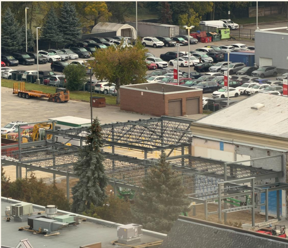
Steel framing beside the church
